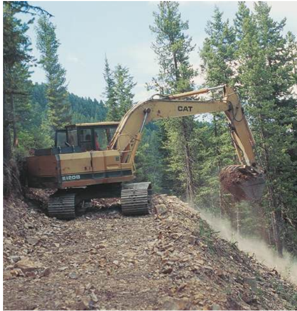
Excavator dismantling the road corridor.
