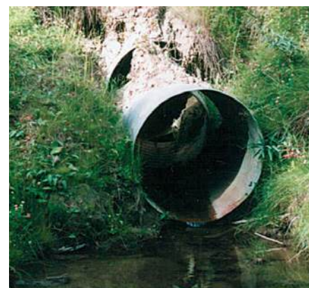
Watch for damaged culverts that need replacement. Repair work should be completed during dry weather.
