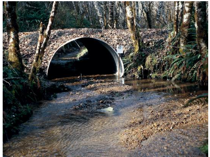
Arch culvert on a low-clearance road, sunk into the streambed to allow for fish passage.
