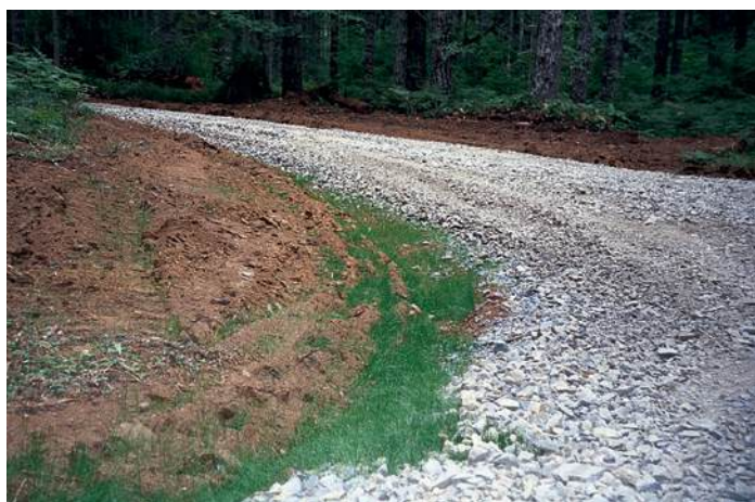
Road surfacing can double the cost of a road. However, gravel roads can provide all-weather access, reduce road maintenance costs and protect water quality by covering the soil with a weather-resistant surface.
