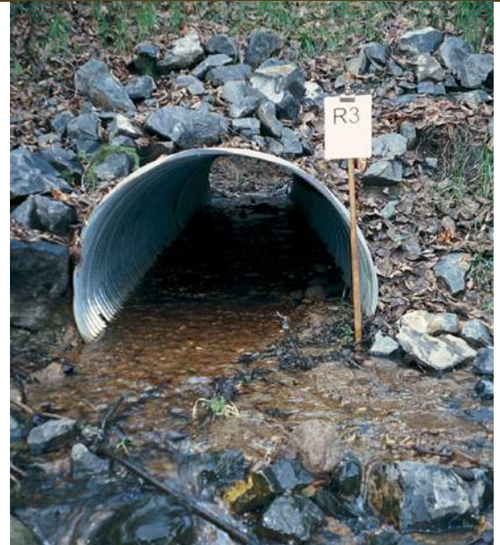
A round galvanized corrugated metal pipe sunk into the streambed to allow for fish passage.
